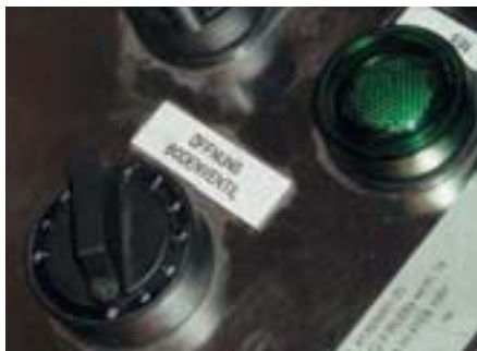
Figure 6: Explosion protected control device for controlling the product release
