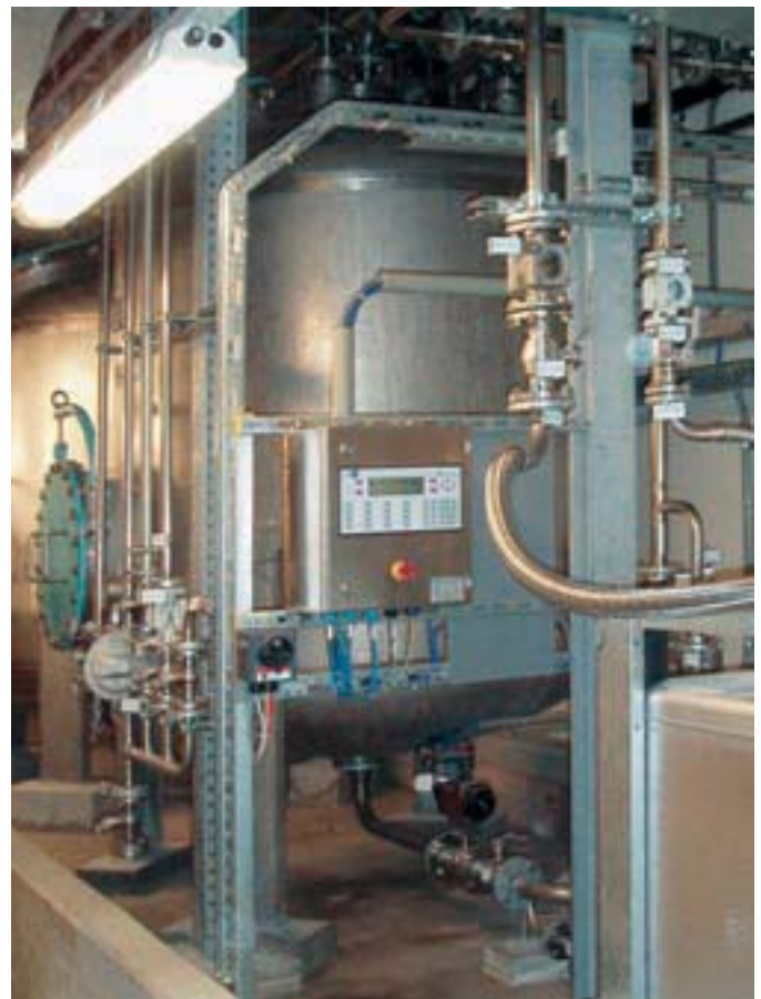
Figure 7: Effluent collecting depot with explosion protected operator display
